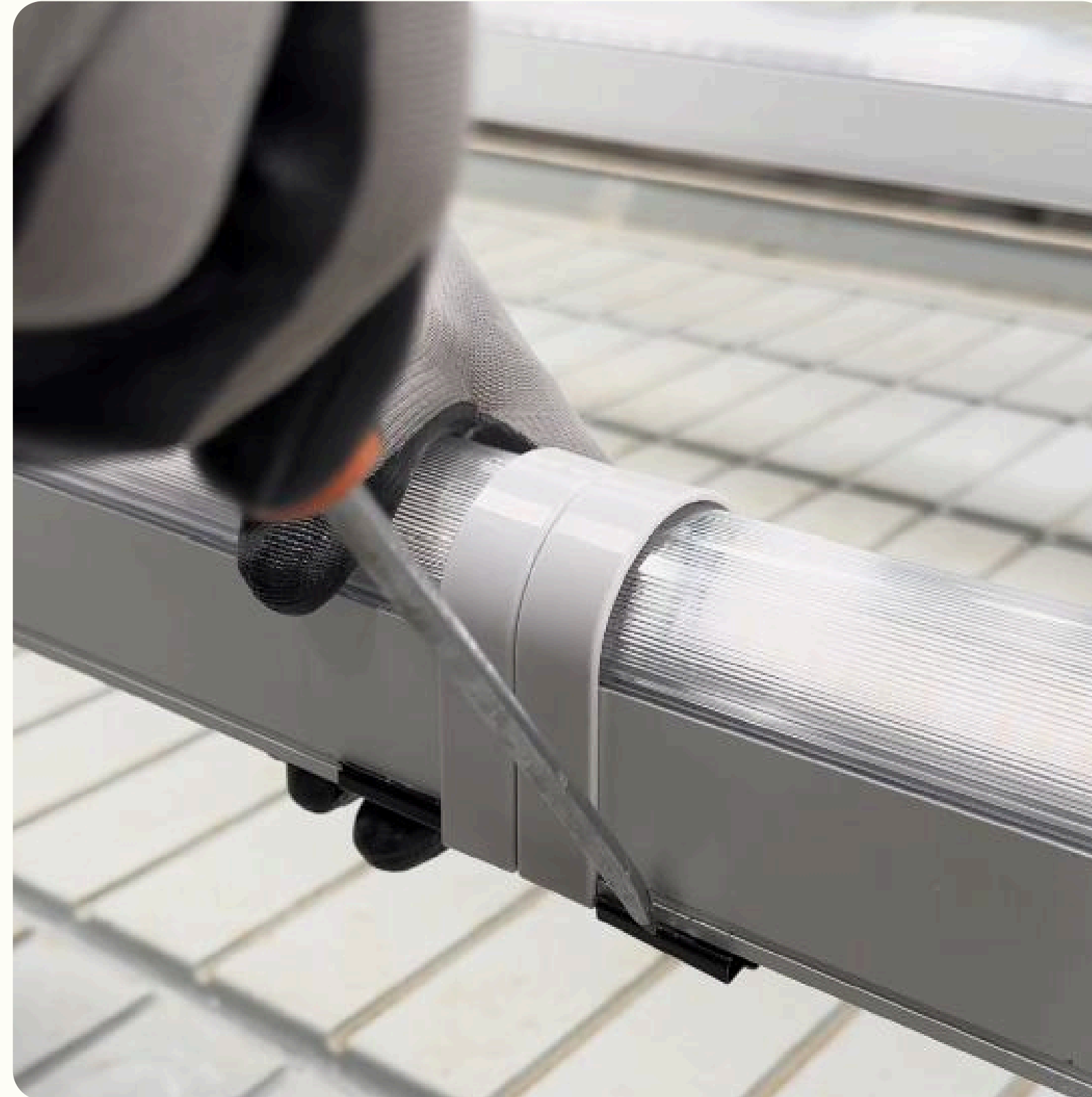
Fig 10. Removal of Interconnection Clips
