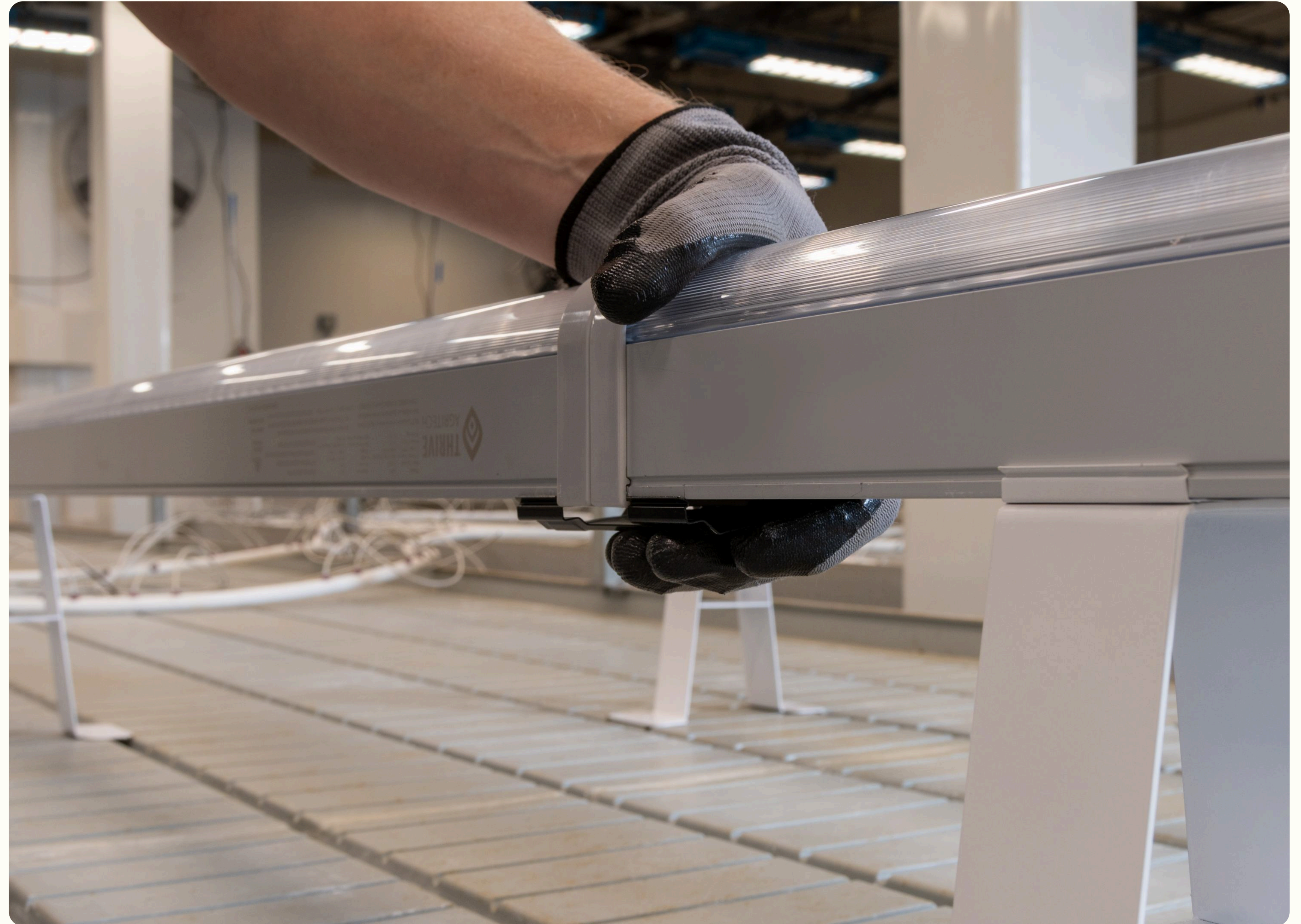
Fig 4. Secure the lights to together with the Interconnection Clip
